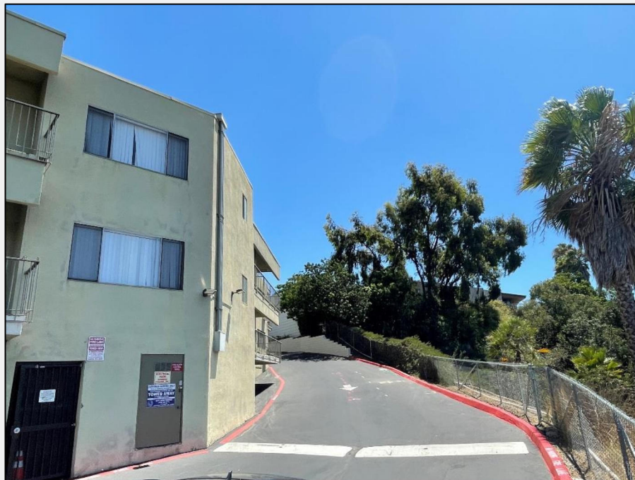
Photograph 14: Overview photograph of the existing setback of structures from the top of slope at the northwestern portion of the Peninsula area. Photograph taken from the northwestern corner of the area facing southeast.
